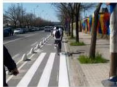
2. Bollards or other low elements separating bike lanes from vehicular lanes with a separate sidewalk for pedestrians
